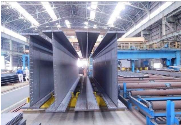
鋼桁の組立て
